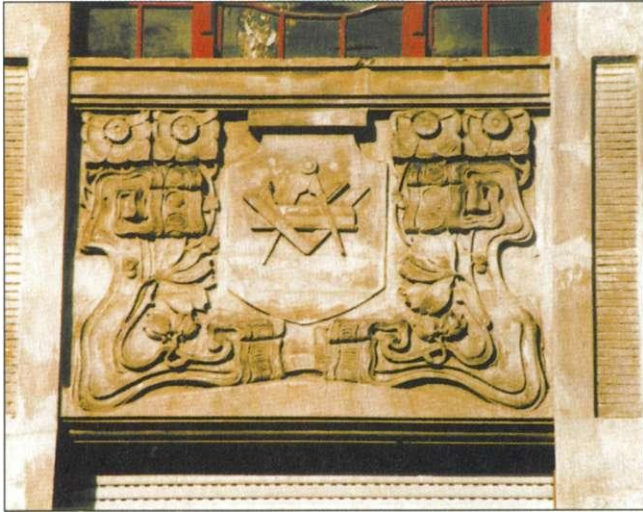
Abb. 197 Alexander-Puschkin-Straße 26, Stuckrelief am Erker
